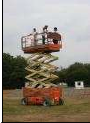
MTA International crew on a scissor lift
